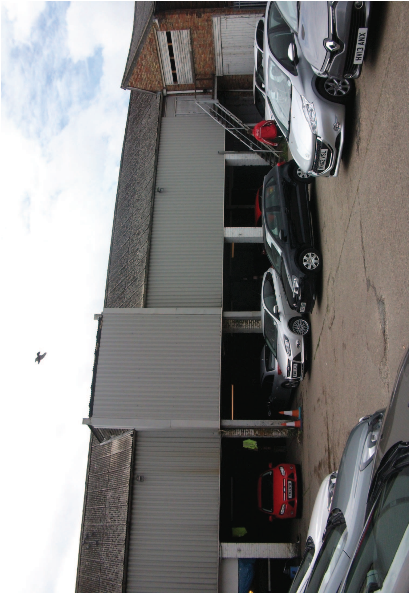
View of existing buildings on the site
